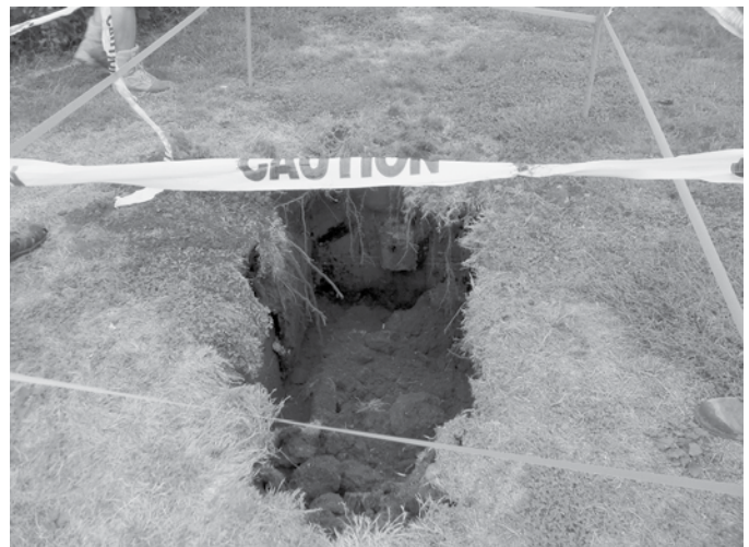
Tank Collapse
